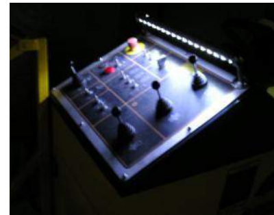
3/ Lighting installed on the control panel of the loader
